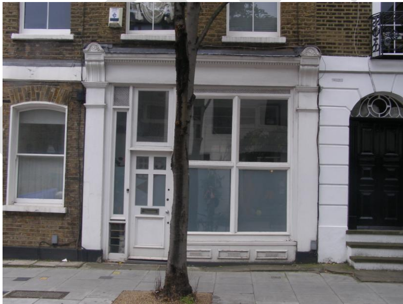
Figure 9: Wintergarden behind retained shopfront – a shop converted to residential, with wintergarden and obscured glass, Islington
