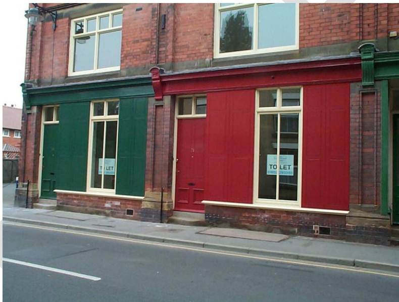
Figure 11: A shopfront converted to residential – solid panels that look like traditional external shopfront shutters, Wem, Herefordshire
